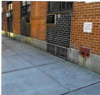
a. Ventilation openings near sidewalk level
