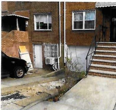
c. Driveway sloping down to converted basement
