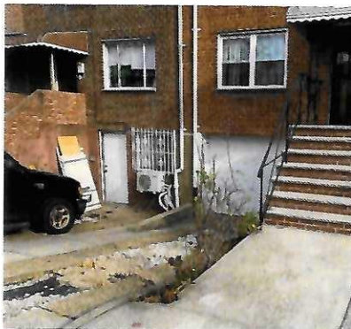
c. Driveway sloping down to converted basement
