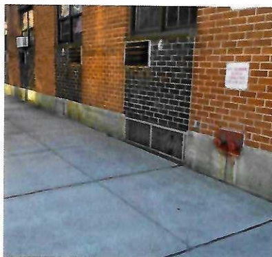
a. Ventilation openings near sidewalk level
