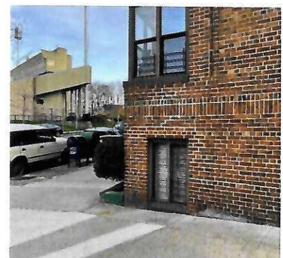
b. Basement window sill near sidewalk level
