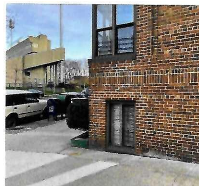
b. Basement window sill near sidewalk level
